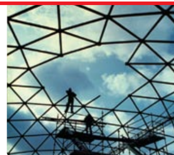
La Géode nears completion. This Buckminster Fulleresque dome, built in Paris in 1985, uses 1,670 steel triangles.
